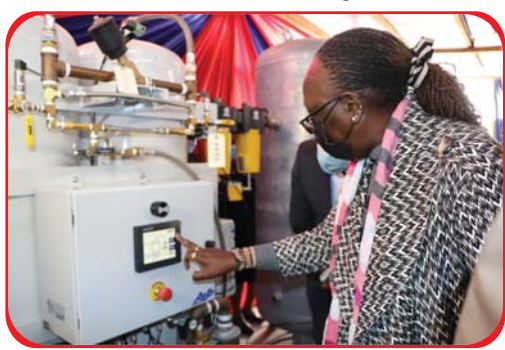
CS Betty Maina switching on the newly commissioned oxygen plant.
